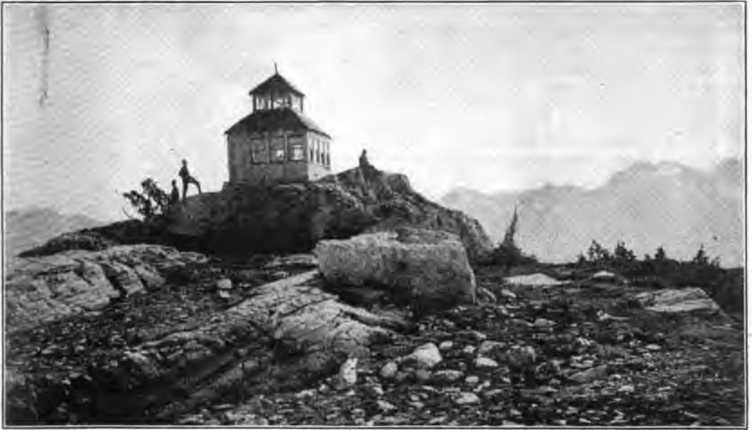
LOOKOUT HOUSE IN THE WASHINGTON NATIONAL FOREST, WASHINGTON
